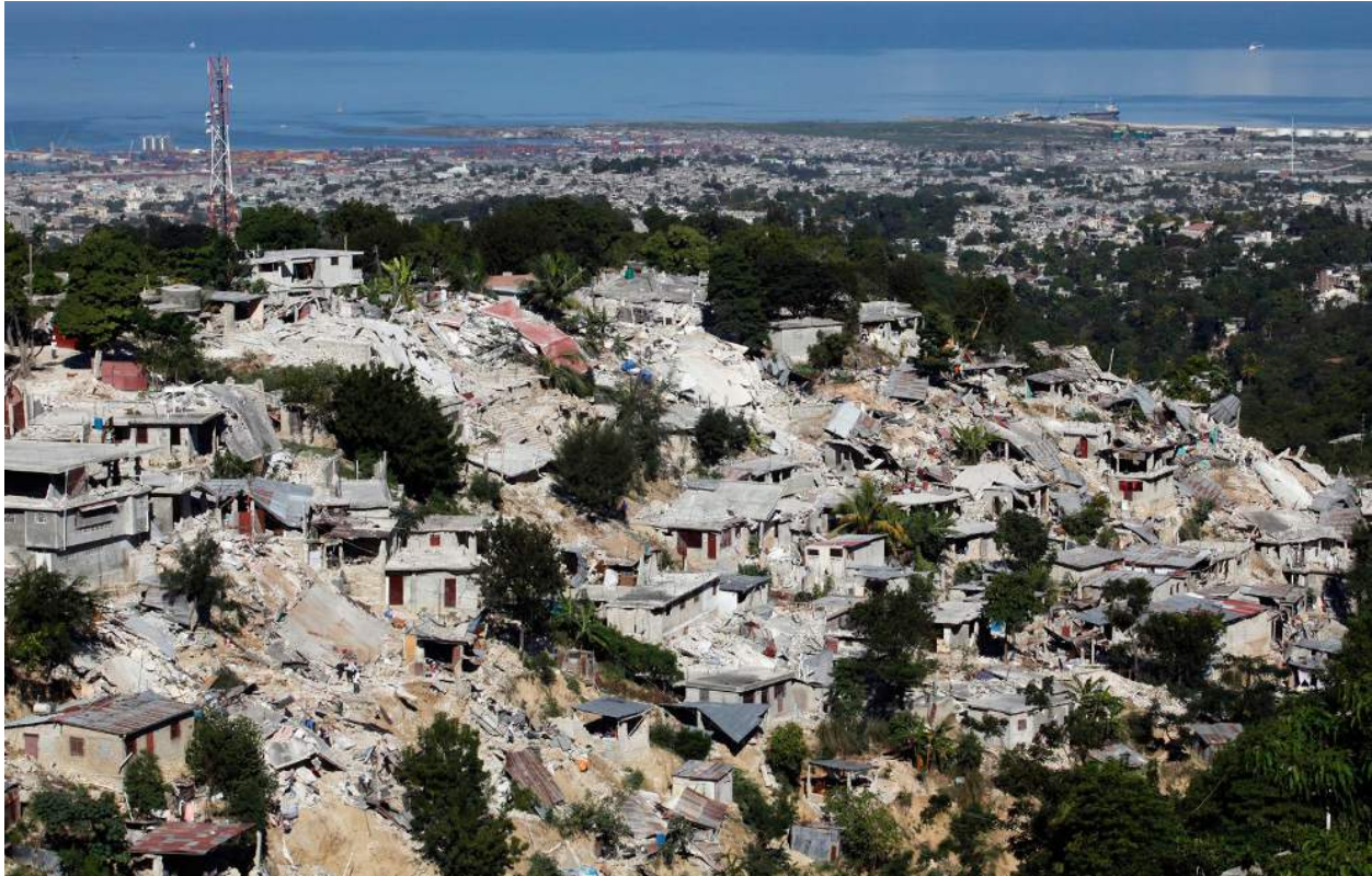
Figure 22h. Chaos on a bedrock hill overlooking Port au Prince. The Bible, geologic and architectural conventional wisdom, and even common sense, suggests that “build ye not a house on sand, but on bedrock.” Here’s a bedrock side hill with no faulting and no indication that the regolith is sliding toward the ocean. There is apparently a complete spectrum of residential construction quality on this side hill. A significant minority of houses appear to be perfectly intact, proving intact was possible. A significant number are completely demolished, proving poor design, materials, or workmanship are at fault. Compare this picture with the Turnagain Heights residential area near Anchorage.
