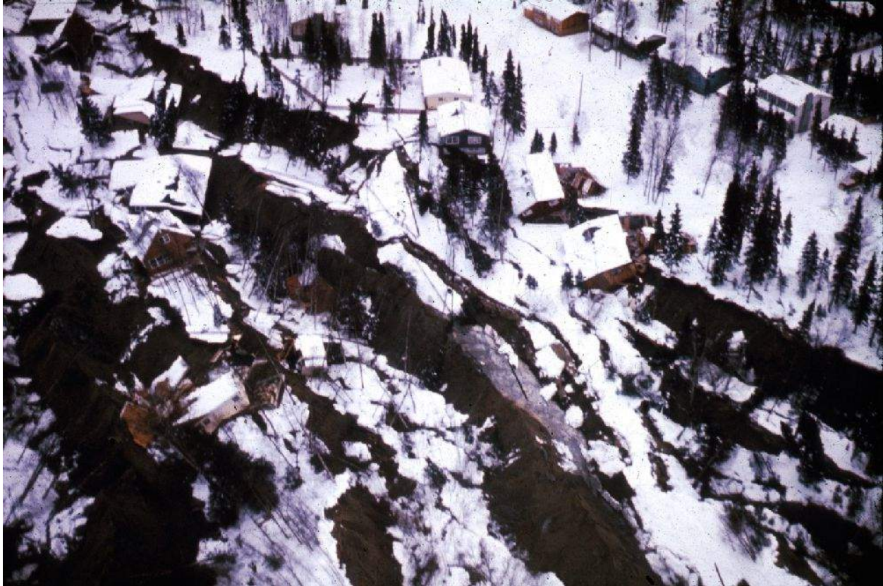
Figure 22g. Turnagain arm, an Anchorage residential area. At first it looks like utter chaos, but look again. Almost all the houses are intact, though tilted, even though the ground has been liquified by the shaking and is flowing toward the adjacent water. Those houses are performing superbly, acting like boats, intact, bobbing on a stormy sea.
