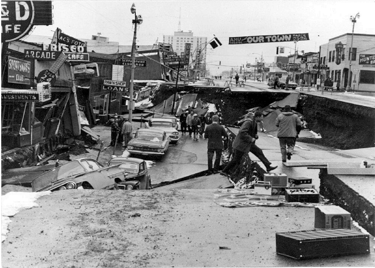
Figur 22a . This picture is characteristic of the business district in Anchorage: There is a one story high normal fault scarp in the foreground, and the whole row of buildings on the other side of the street, and the high rise in the background, are intact. There is not a single instance in this picture of a higher floor collapsing on a lower one.
